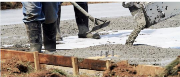
Carpentry – Concrete, Finish Carpentry, Framing, Tilt-up
