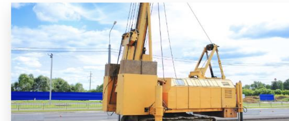
Carpentry – Pile Driver
